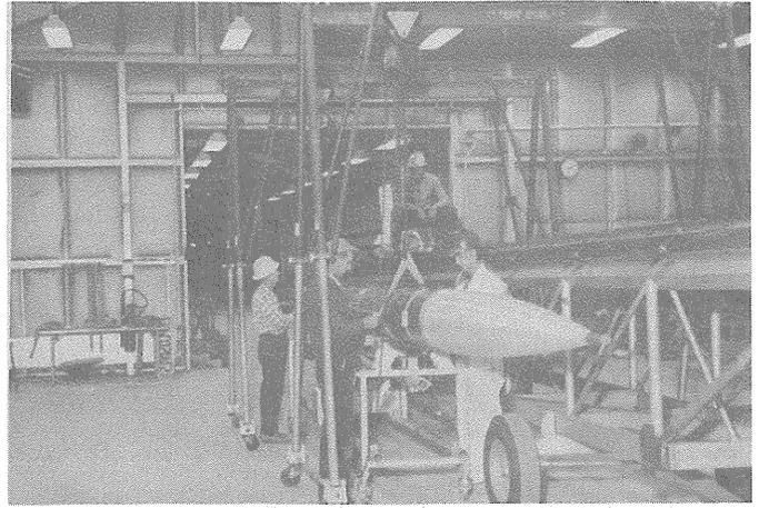
**(e) Transfer of sounding rocket from assembly dolly to launch rail dolly, Step 1.**
