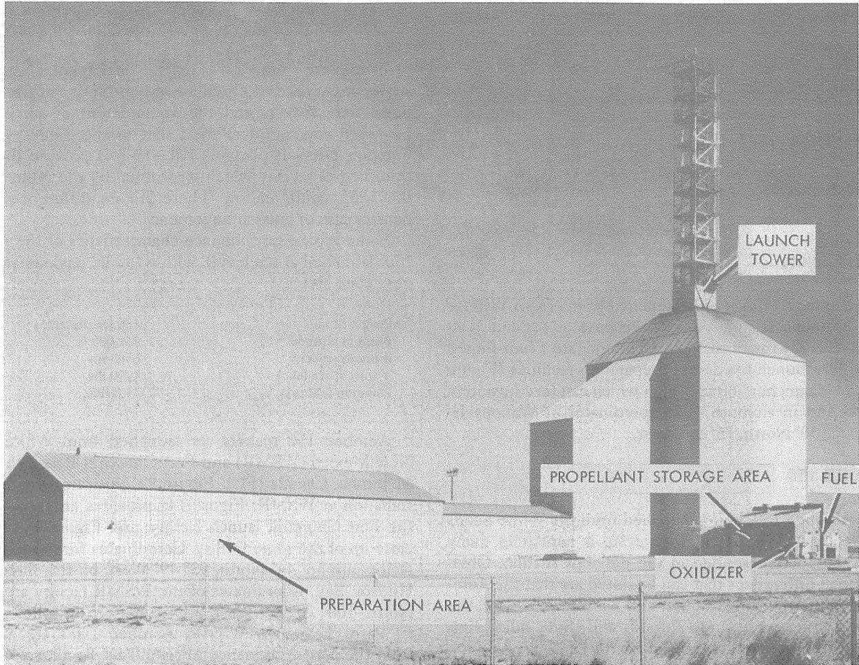
**Figure 8 - Aerobee launch facility at Wallops Island.**
